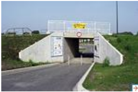
Road- and Bridge Construction
